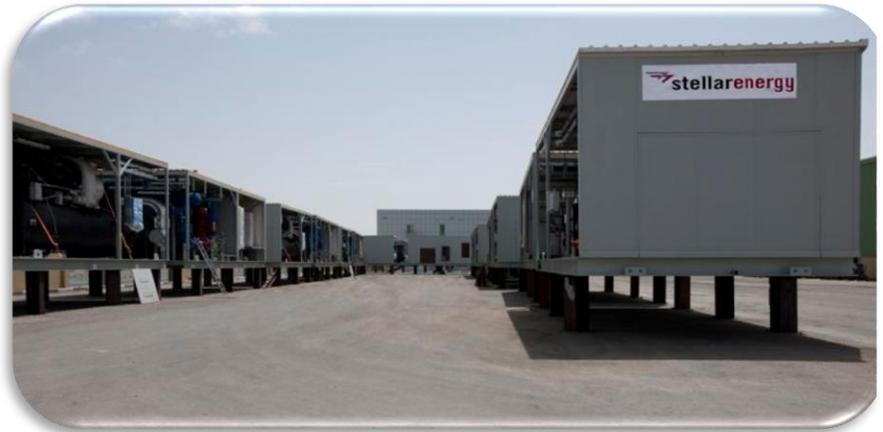
Stellar Energy delivered 16 water-cooled modules for the turbine inlet air chilling system that will produce a total of 92,000 tons of chilling in order to increase efficiency and power output of the Qurayah IPP.
