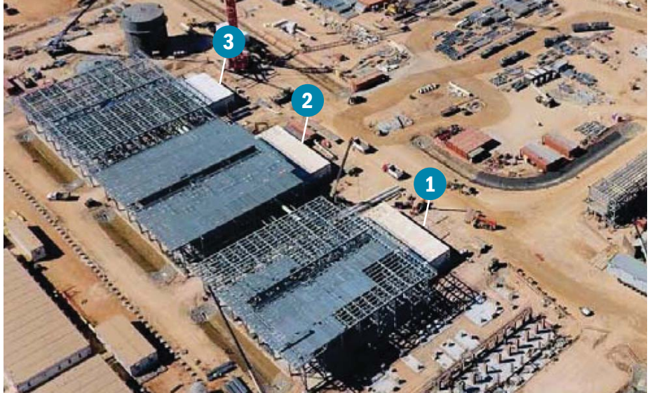
Pictured, top left: The three chiller plants consist of 18 factory-built modules that were custom-designed, pre-engineered and fabricated in a controlled, ISO-certified environment. Modular fabrication enabled a 50% reduction in construction time. Bottom left: Packaged in an enclosed, climate-controlled skid, the modules were pre-piped, wired, tested and shipped to site. Right: All three modular chiller plants (labeled in the photo above) were reassembled on site (image source: www.cheniere.com ).
